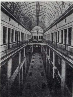
Light roofing of the Golofeev Passazh (Arcade) in Moscow. A photo of 1913
