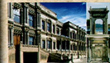
NEW ÇIRAGAN PALACE The palace, built by Sultan Abdülhamid II was designed by the Armenian palace architect Nigârîsâr Balyan and constructed by his brothers Tarkhan and Nigârîsâr Balyan between 1883 and 1887. The inner walls and the roof were made of wood, the outer walls of colorful marble. A beautiful marble bridge connects the palace to the Yıldız Palace on the hill behind Sultan Abdülhamid II. It is one of the gems of Çırağan in Yıldız. It is a very high garden wall protects the palace from the outer world. It is located on the European shore of the Bosphorus.
